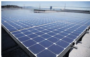
The Exploratorium has 5,874 solar panels that will provide 1.3 megawatts of electricity.
